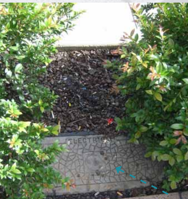
Garden bed and access point to underground services.
